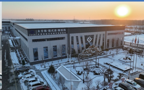
Mobile cabin production base
