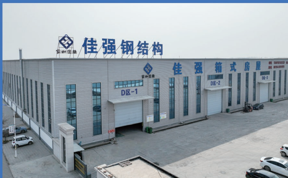
Steel structure production base
